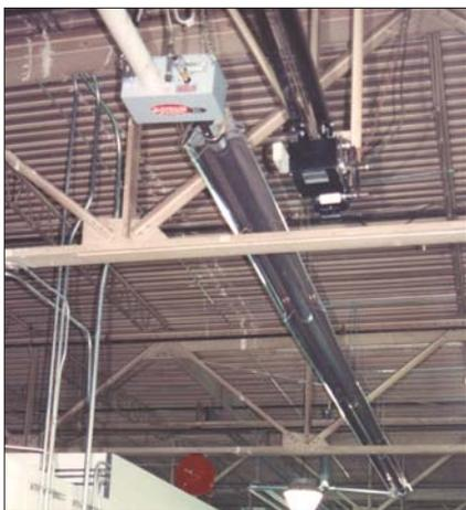
The inside of the test site, representing a typical industrial building and showing the RE-VERBER-RAY Two-Stage *HL Series*. This heating system objectively documented a minimum of 12% additional energy savings - and a 35% reduction in "On and Off Cycles" - when compared to a single input system.
