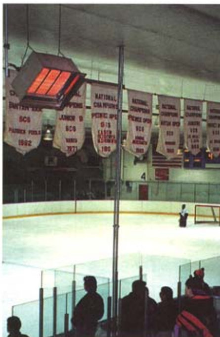
Gas-fired infrared heaters can provide heat that is absorbed by people, flooring, and seating, and directed to avoid heating the delicate ice surfaces.
